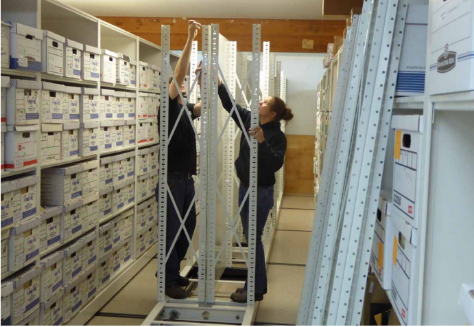
The contractor's crew installs the Borroughs carriage of mobile shelving on the west side of the lower floor.
