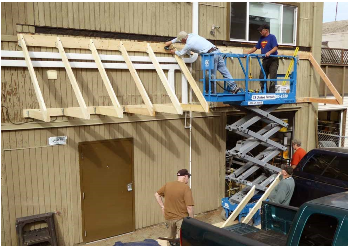
On the south side of the Archive, Bill Petryk secures an awning frame from the lift as the rest of the construction crew are ready for the next frame.
