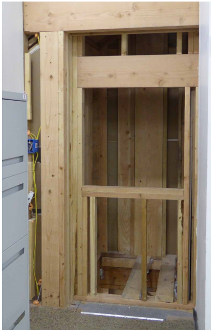
The hoistway framing on the Main floor of PNRA's new Box-Lift system.
