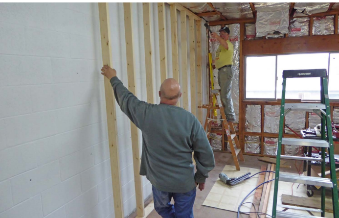
Volunteers, Don Larson & Rod Olson install the wall framing to fur out the east wall of the upper floor.
