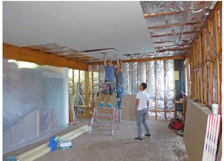
The contractor's crew hanging drywall on the ceiling of the Upper Floor. All the Archive items were moved to the center section on the left during the work.
