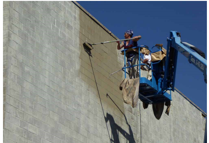
An elastomeric coating being applied to seal the east wall of the Archive after the old paint was removed.
