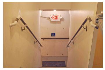
Steel handrails were fabricated and installed on all three walls of the stairs to the lower floor. Also note the lighted and tactile exit signs at the bottom of the stairs.
