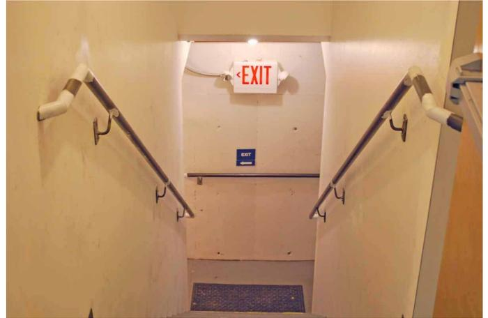
*Steel handrails were fabricated and installed on all three walls of the stairs to the lower floor. Also note the lighted and tactile exit signs at the bottom of the stairs.*
