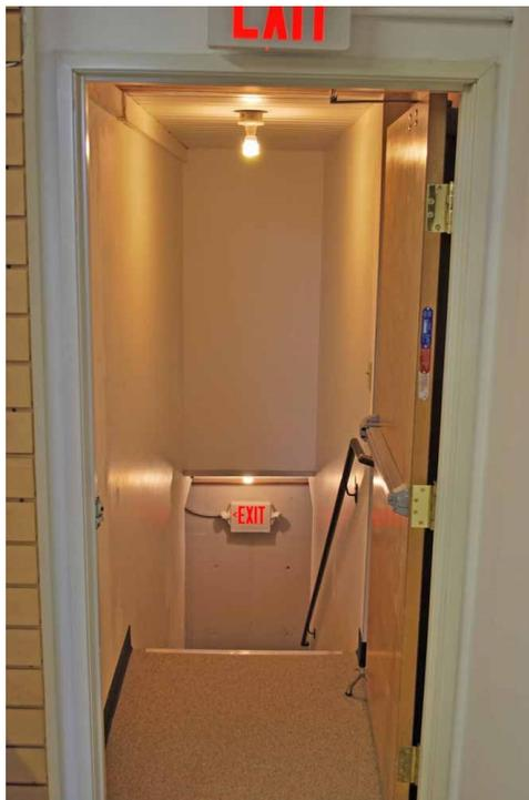
*New overhead light, exit lights and new vinyl installed in the stairwell to the lower floor.*
